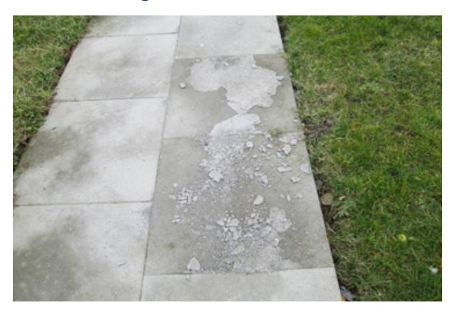
Rock salt is corrosive and can damage both natural stone and concrete paving slabs, causing the surface to break up. Concrete paving is particularly vulnerable to the corrosive effects of rock salt and most paving manufacturers warn against the use of rock salt. Unfortunately, corrosion caused by rock salt is irreparable, but the damage should not worsen if no more rock salt is used.
