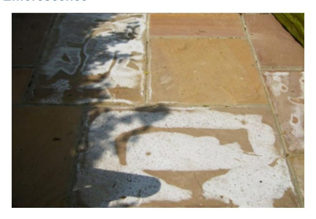
Efflorescence, also known as 'lime blooming', affects concrete paving and is caused by the reaction between cement and water, seen as darker circular spots on the paving. The phenomenon has a similar appearance to 'void bedding' but it is not caused be incorrect installation. Efflorescence is a natural phenomenon and not an issue with the paving slabs.
