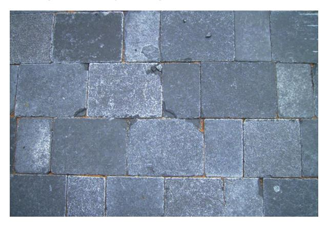
Paving slabs, regardless of the material, should be installed with a gap between each slab. Paving slabs should not butt up against each other, this does not allow the slabs to expand and contract with changes in temperature, and it will not be possible to point the slabs correctly. Common issues associated with butt jointing include:
