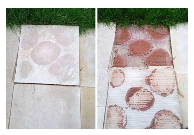
All paving slabs, regardless of materials, should be laid on a full bed of mortar. Under no circumstances should paving slabs be void bedded. Void bedding, also referred to as "dot & dab" or "the 5-spot method", leaves gaps under the paving slabs and does not fully support them. Void bedding may cause these common issues:
