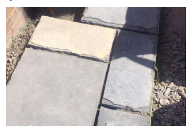
It is important to lay paving slabs with the correct surface facing upwards. For concrete slabs, identifying the flat unfinished underside should easy but for natural stone slabs this can be more difficult.
